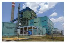
Photo of Coal-fired power plant near Cirebon (West Java), currently the installed capacity is 650 MW and the production of flared CO2 is about 4 mio. Tonnes per year. In 2022, unit-2 will be on stream with additional capacity of 1,000 MW.
